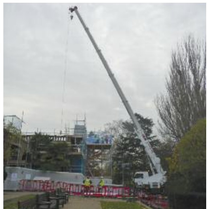
Work on the Belvedere roof
