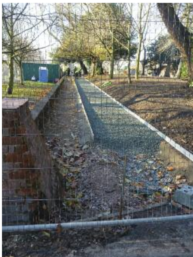
Foundations for the access ramp
